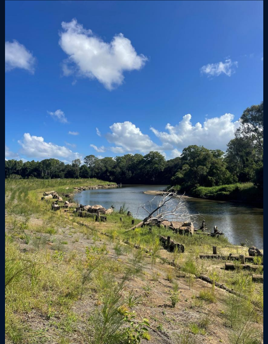
Riverbank Restoration Project, Unitywater, Sunshine Coast, Australia
